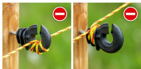
Do not wind the wire on the insulator!
